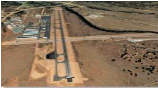
Truckee Airport facing NW
