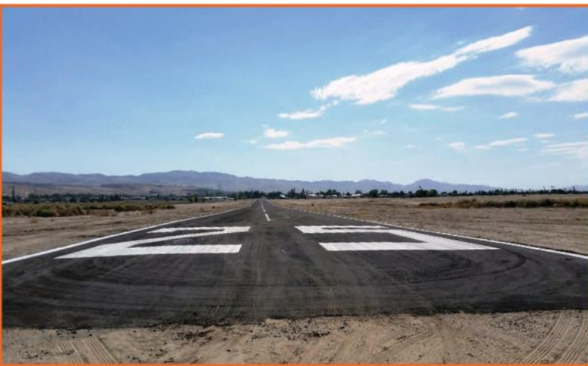
Completed Slurry Seal and Restriped Marking
